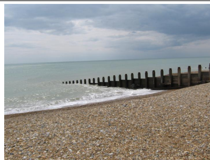
HAZARD – groynes, risk of falling
